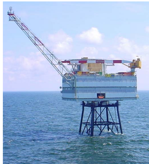
Figure 2: Q4-C Gas production platform
